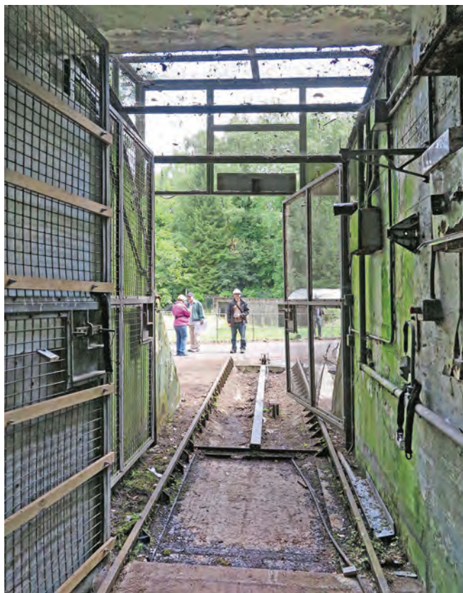
Looking out from the emergency exit. This is also used for taking equipment in and out of the bunker on a trolley which travels on rails straddling the stairs.
